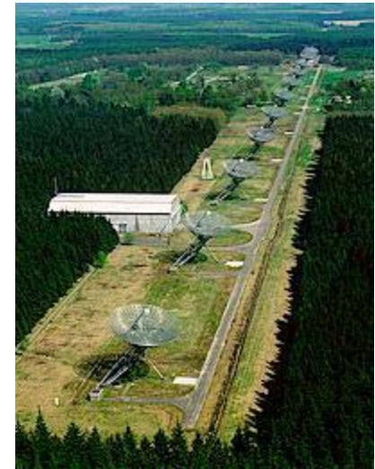
Line array of directional sensors Westerbork Synthesis Array Radio Telescope, (WSRT) the Netherlands.
