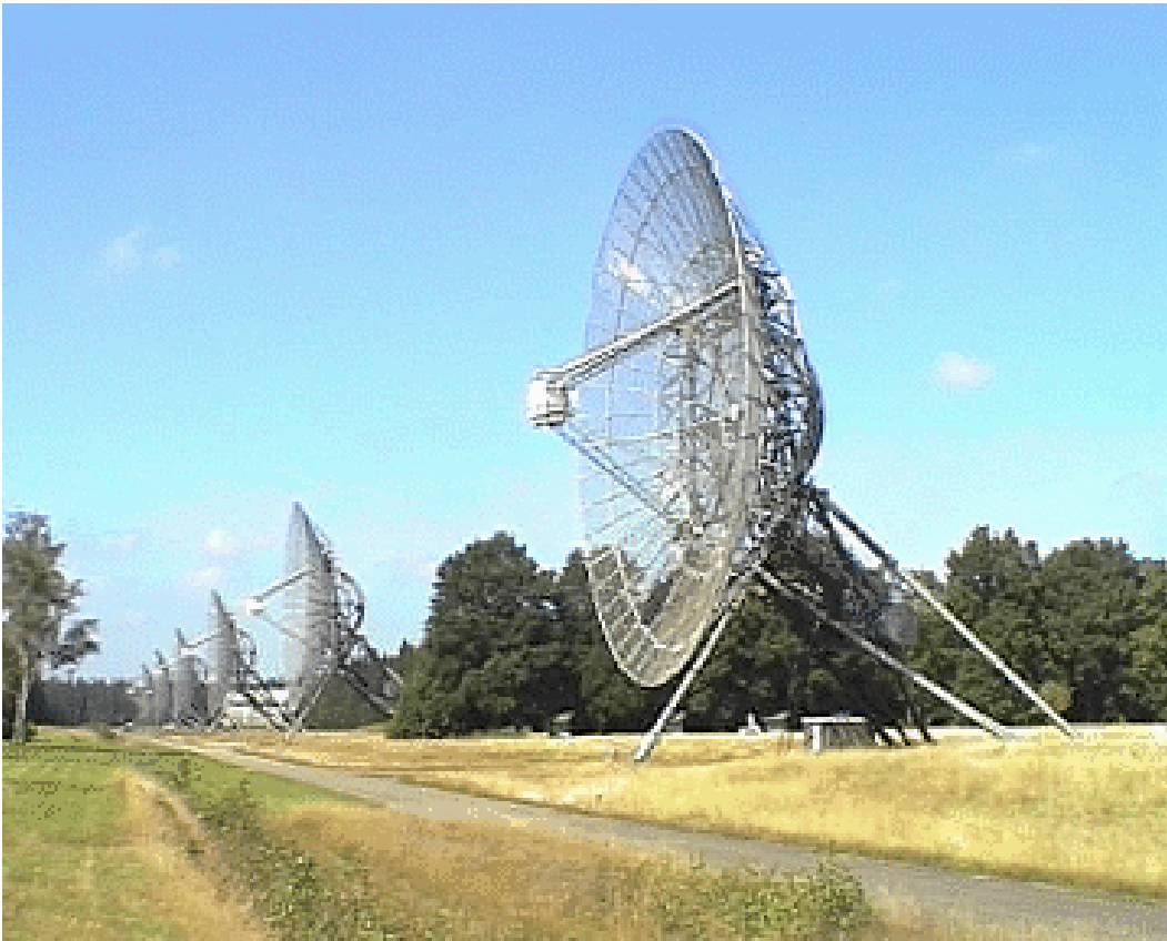
Line array of directional sensors Westerbork Synthesis Array Radio Telescope, (WSRT) the Netherlands.
